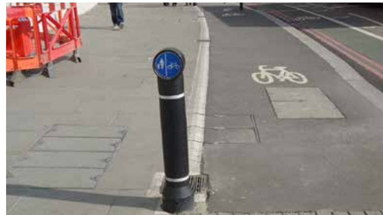
Example of shared footway / cycleway with delineation
